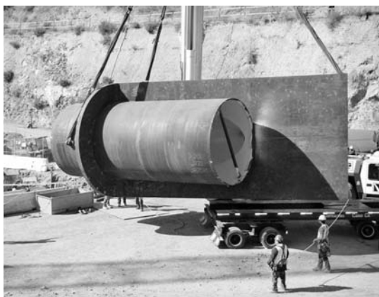
A crane prepares to lower the large Y-shaped pipe.
