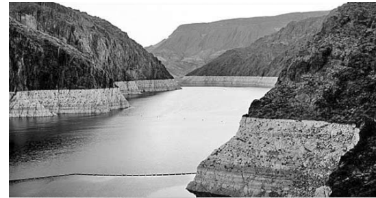
The "bathtub ring" around Lake Mead measures an unprecedented 10 stories high, providing vivid evidence of drought in the Colorado River system.
