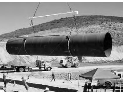
Large 50-foot-long pipe sections will create the San Vicente Pipeline.
