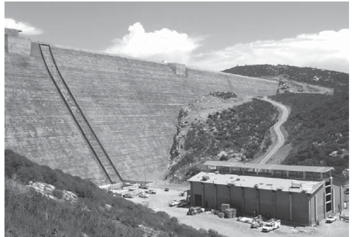
The Olivenhain Dam serves as an impressive background to the Olivenhain Pump Station.
