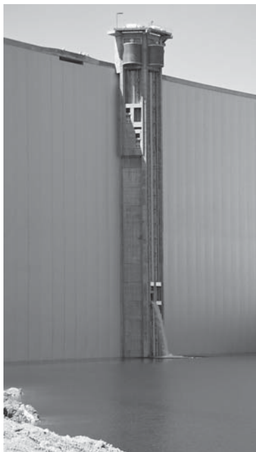
Imported water cascades into the Olivenhain Reservoir.
