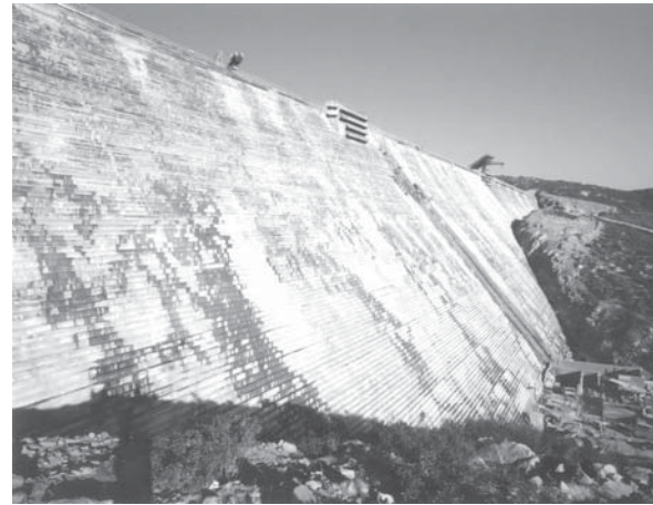
The Olivenhain Dam at 318 feet high and 2,552 feet long.
